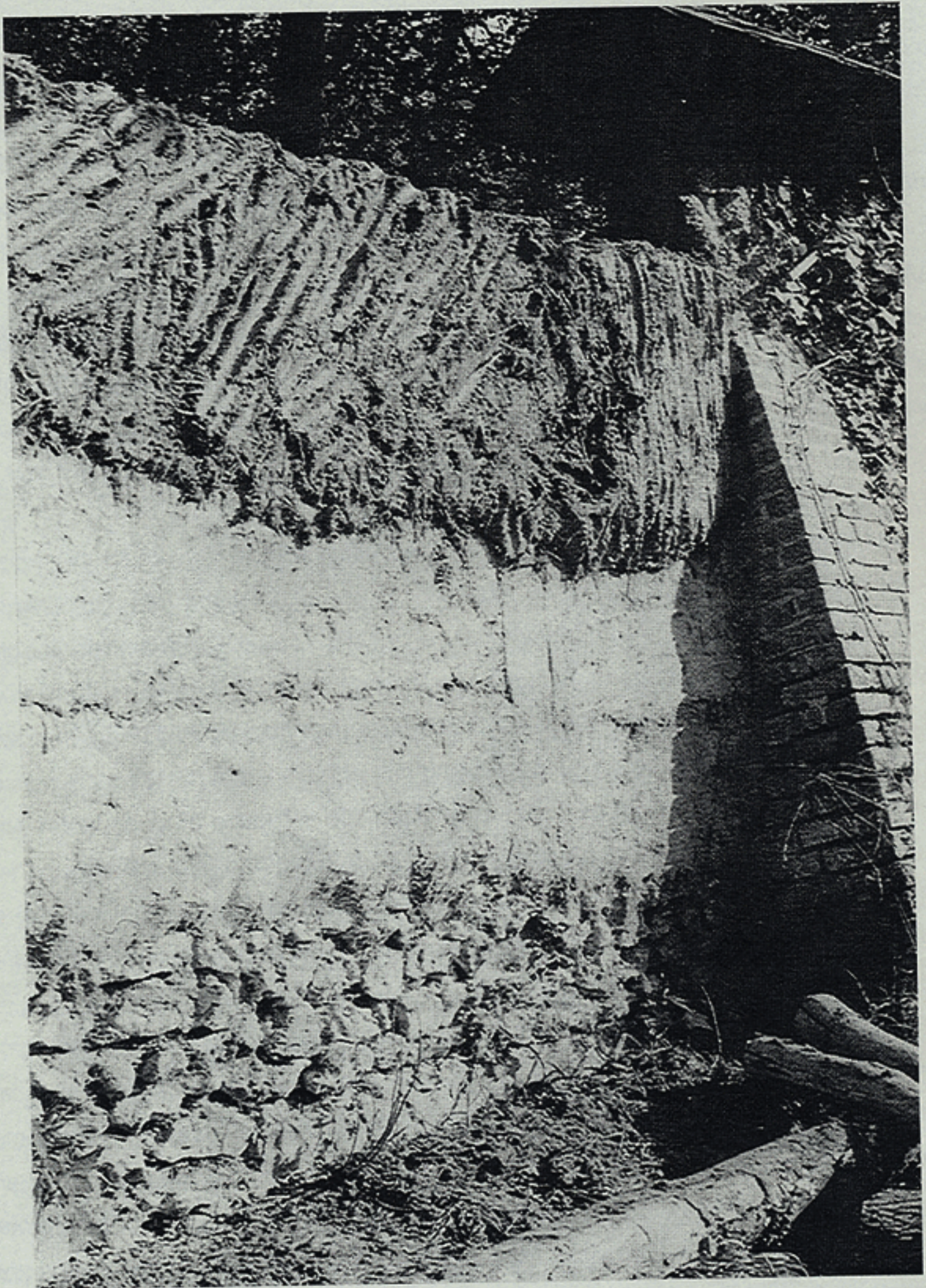
Re-construction of cob boundary wall in Eure, Normandy.
