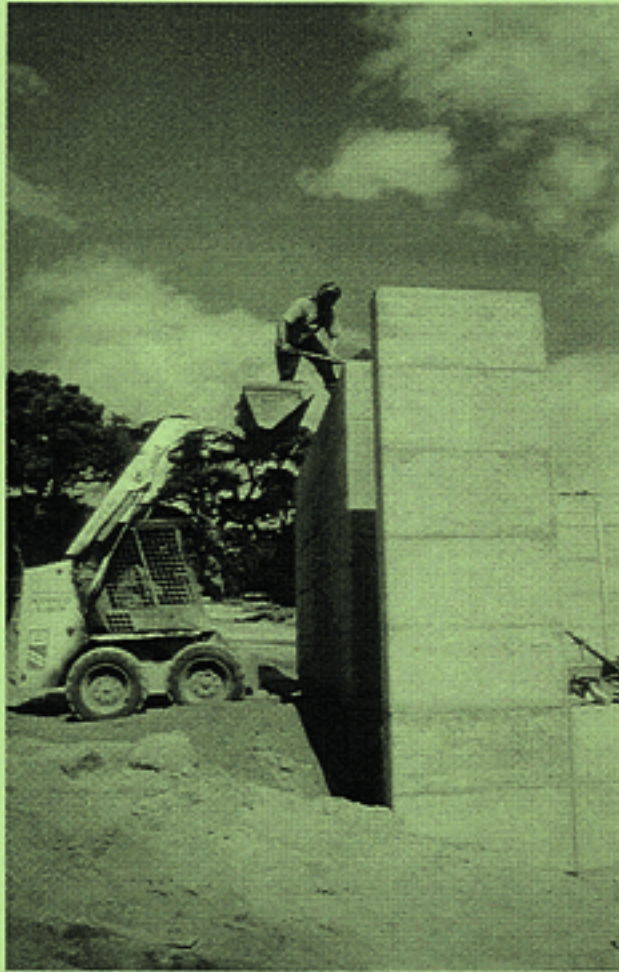
Rammed earth wall under construction.
