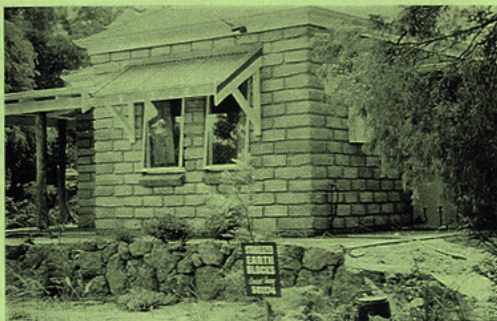
Stabilised earth block house near Bunbury.
