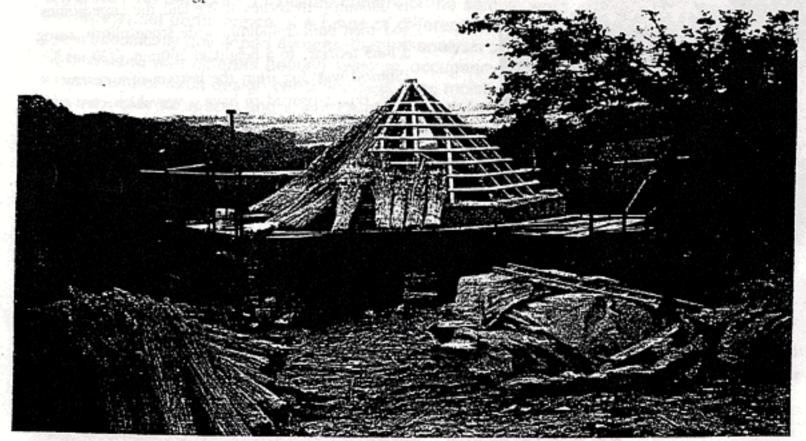
After discussion with the thatcher ( Charles Chalcraft ) it was decided to put a softwood ringbeam in, to make a fixing for the secondary timbers and the first course of thatch. The thatch is now virtually complete and the final pitch is approximately 55 degrees. We have reclaimed some cobbles which will be set into the floor ( in some, hopefully, interesting pattern ). The oak window frames and oak plank door will be fitted at a later date.
