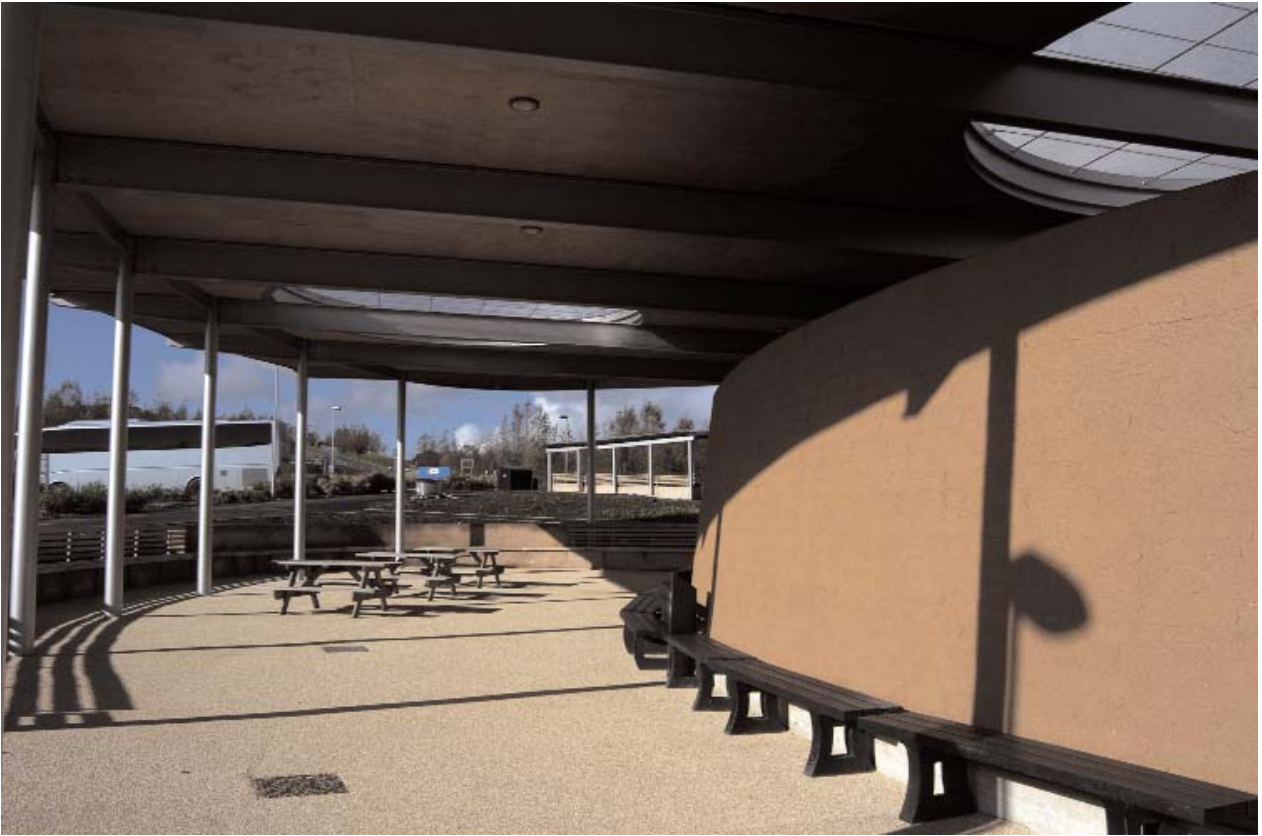
Seived earth and Hemp exterior plaster
