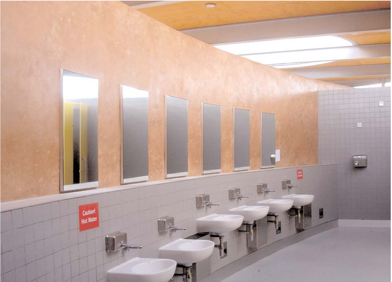
Earth/Lime interior plaster finished with beeswax
