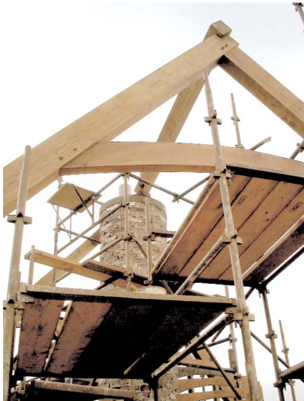
Cadhay roof structure
