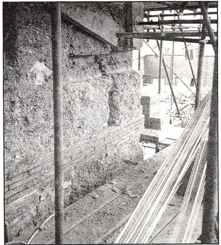
Crack stitching with cob tiles: Town Farm, Gittisham.
