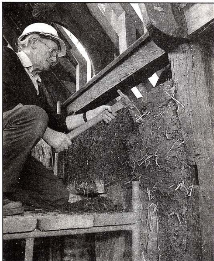
Paring back new cob inserted as a repair at Bowhill, Exeter.
