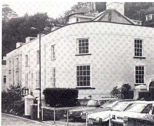
Large 18th century cob warehouse at Shaldon, converted into seaside villas around 1830.
