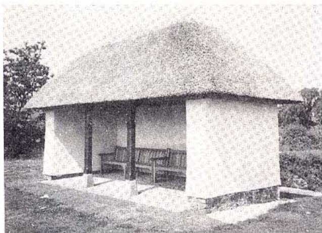
Cob shelter at Starcross built by Teignbridge District Council in 1989.
